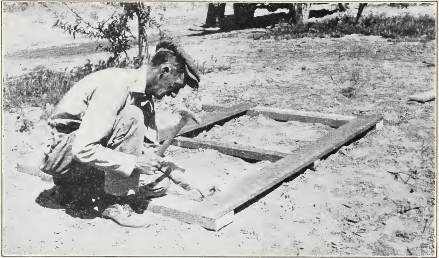
Fig. 6—Squaring up and starting the side-wall form.
